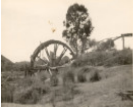
B0709 Water Wheel Timber Water Race Wandiligong nr Bright
