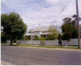
SL 350 - House, 26 Skene Street, STAWELL
