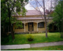
SL 353 - House, 29 Skene Street, STAWELL
