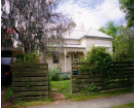
SL 354 - House, 31 Skene Street, STAWELL
