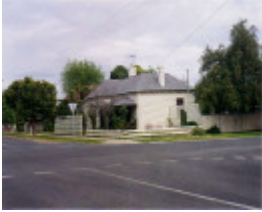
SL 356 - House, 34 Skene Street, STAWELL
