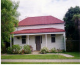
SL 358 - House, 36 Skene Street, STAWELL
