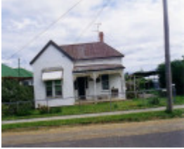
SL 362 - House, 44 Skene Street, STAWELL
