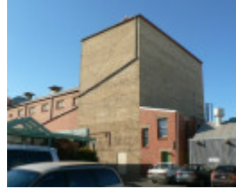
Horsham Theatre rear view of fly tower 2009
