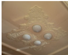
Horsham Theatre detail of ceiling 2009
