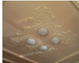
Horsham Theatre detail of ceiling 2009
