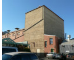
Horsham Theatre rear view of fly tower 2009
