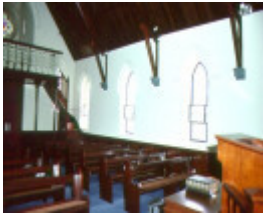
St Johns Streatham Interior September 2000
