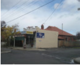
Shop and attached dwelling at 69/71 Chomley Street.
