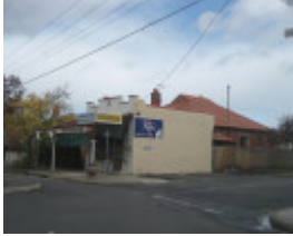
Shop and attached dwelling at 69/71 Chomley Street.
