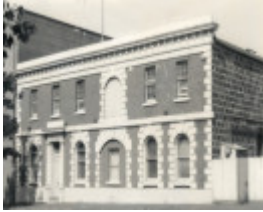
B1784 Stores Brougham St Geelong
