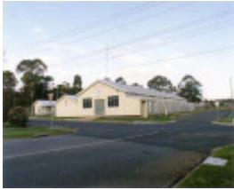
SL 372 - Army Drill Hall, Sloane Street (corner St George Street), STAWELL
