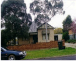
SL 378 - House, 55 Smith Street, STAWELL
