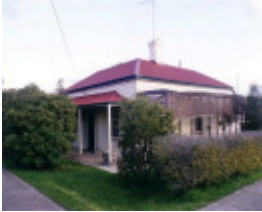
SL 380 - House, 8 St George Street (corner Florence Street), STAWELL
