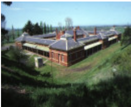
1 caloola former caloola centre the avenue sunbury rear view of property layout apr1991
