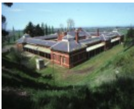
1 caloola former caloola centre the avenue sunbury rear view of property layout apr1991
