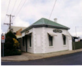
SL 385 - Shop, Victoria Place corner Church Street, STAWELL
