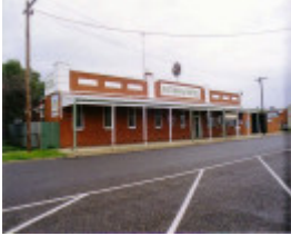
SL 393 - National Hotel, 16 Wakeham Street, STAWELL
