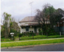
SL 394 - House, 18 Wakeham Street, STAWELL
