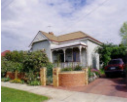
SL 396 - House, 36 Wakeham Street, STAWELL
