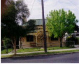
SL 403 - House, 59 Wakeham Street, STAWELL
