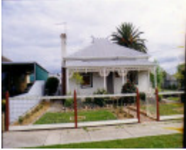
SL 404 - House, 60 Wakeham Street, STAWELL
