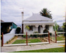
SL 404 - House, 60 Wakeham Street, STAWELL
