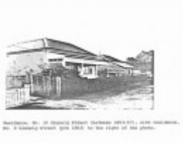
Residence, 8 Glenelg Street to the right of the photo
