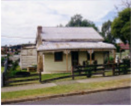
SL 406 - House. 77 Wakeham Street, STAWELL
