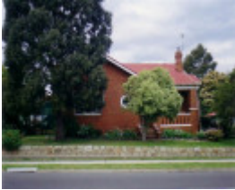
SL 407 - House, Walker Street (corner Darlington Road), STAWELL
