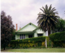
SL 408 - House, 3 Walker Street, STAWELL
