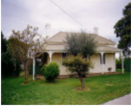
SL 409 - House, 10 Walker Street, STAWELL
