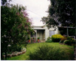
SL 410 - House, 14 Walker Street, STAWELL
