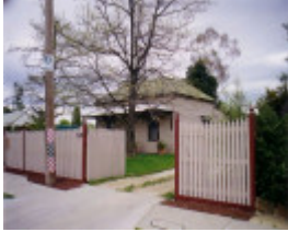
SL 411 - House, 16 Walker Street, STAWELL
