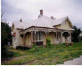
SL 412 - House, 20 Walker Street, STAWELL
