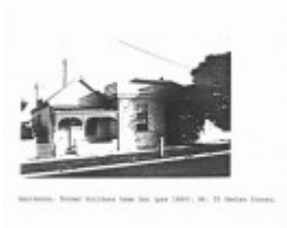
Residence; 25 Gawler Street
