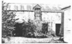
Stone stables (c.1900) in the rear of No. 21 Hurd Street.
