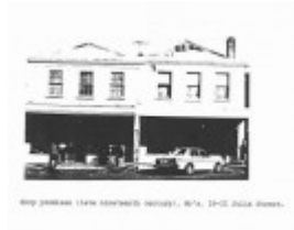
Shop Premises, 19-21 Julia Street
