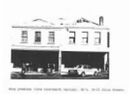
Shop Premises, 19-21 Julia Street
