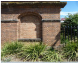
H1673 WATER TOWER LHA 2015 2.JPG
