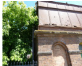
H1673 WATER TOWER LHA 2015 3.JPG
