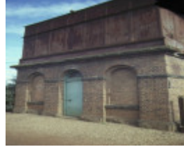
1 water tower sunbury railway station sunbury front detail sep1984
