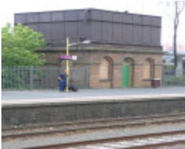
WATER TOWER SOHE 2008
