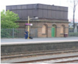
WATER TOWER SOHE 2008
