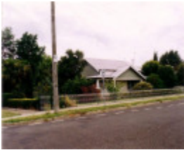
SL 418 - House, Former 'Belmont' College, 6 Wimmera Street, STAWELL
