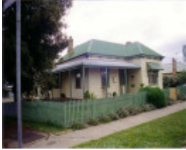
SL 422 - House, 14 Wimmera Street, STAWELL
