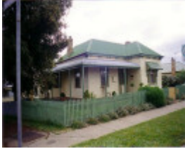
SL 422 - House, 14 Wimmera Street, STAWELL
