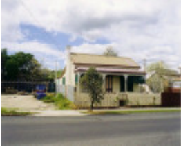
SL 423 - House, 37 Wimmera Street, STAWELL
