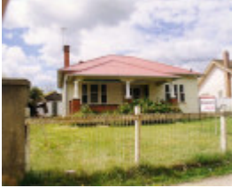
SL 425 - House, 43 Wimmera Street, STAWELL
