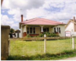
SL 425 - House, 43 Wimmera Street, STAWELL
