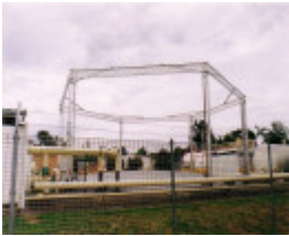
SL 426 - Stawell Gas Holder, 47-49 Wimmera Street, STAWELL
