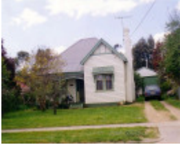
SL 427 - House, 53 Wimmera Street, STAWELL
