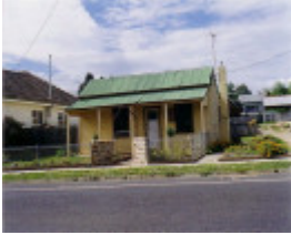
SL 429 - House, 65 Wimmera Street, STAWELL
