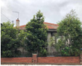
51 Banole Avenue, Prahran
