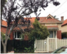
34-36 Banole Avenue, Prahran
