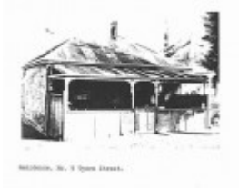
Residence, 9 Tyers Street
