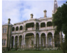
1 rupertswood macedon street sunbury front view detail of lace
