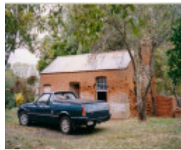
SM 17c - Kitchen building
