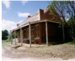
SM 17b - Store prior to renovation
