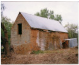
SM 17d - Stables building
