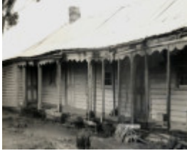
113391 B1694 Glynwylln Campbells Bridge nr Stawell
