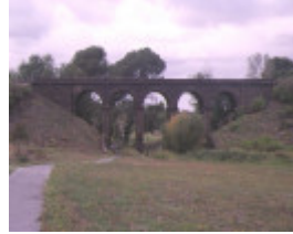
1 rail bridge over kismet creek sunbury side view jun1984
