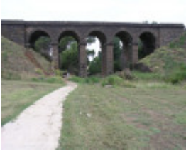
RAIL BRIDGE SOHE 2008
