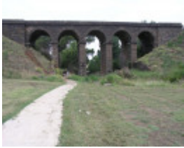
RAIL BRIDGE SOHE 2008
