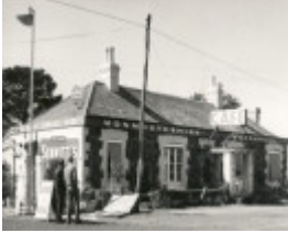
B1260 Monmouthshire Hotel Calder Hwy Diggers Rest
