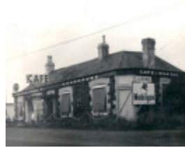
B1260 Monmaoushire Hotel Diggers Rest
