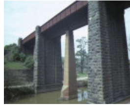
1 rail bridge over jackson's creek sunbury side elevation sep 84
