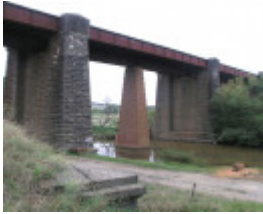
RAIL BRIDGE SOHE 2008
