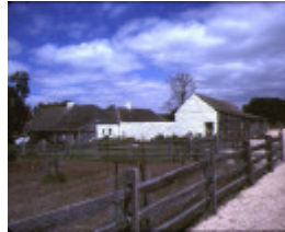
1 emu bottom racecourse road sunbury side view with fencing
